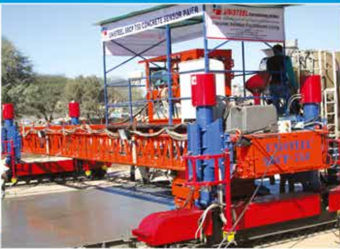
Working on Track Chain SRCP-750
