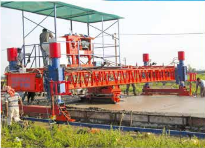
Working on Rail SRCP-720
